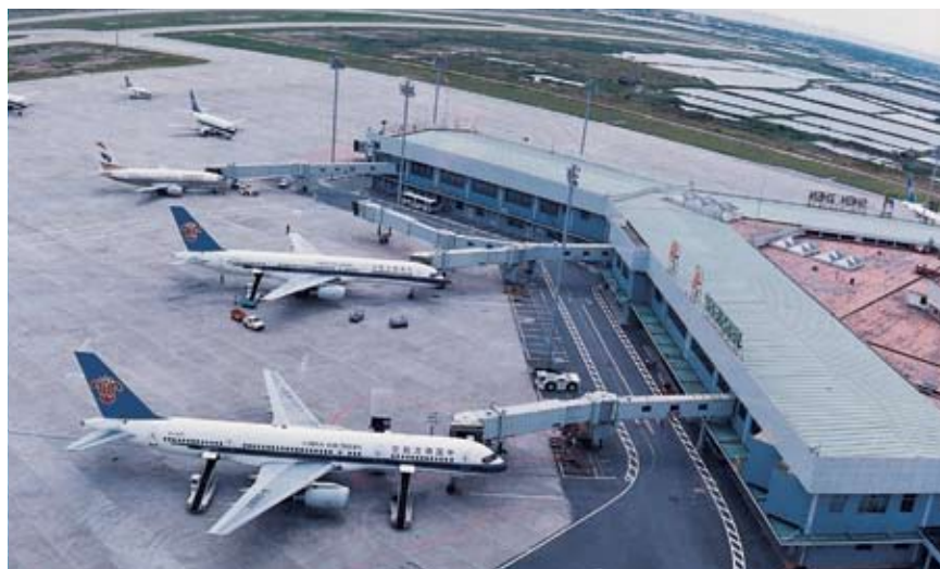
Shenzhen Airport: co-ordination with Hong Kong is critical
