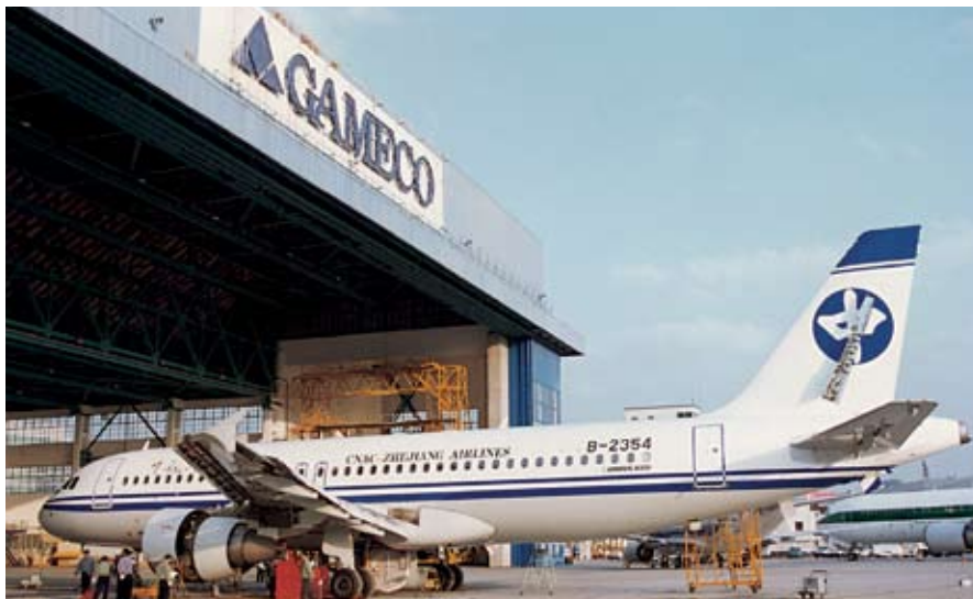
GAMECO's four bay hangar at the New Baiyun International Airport will be the biggest in China
